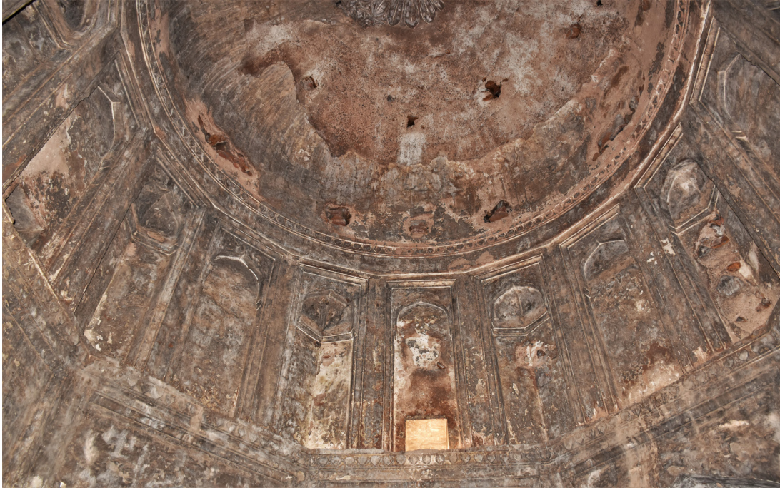
Figure 9: Upper Arch Netting
